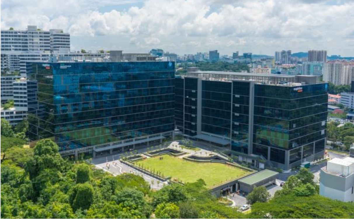
BTS facility for HP at Depot Close by Mapletree Industrial Trust
